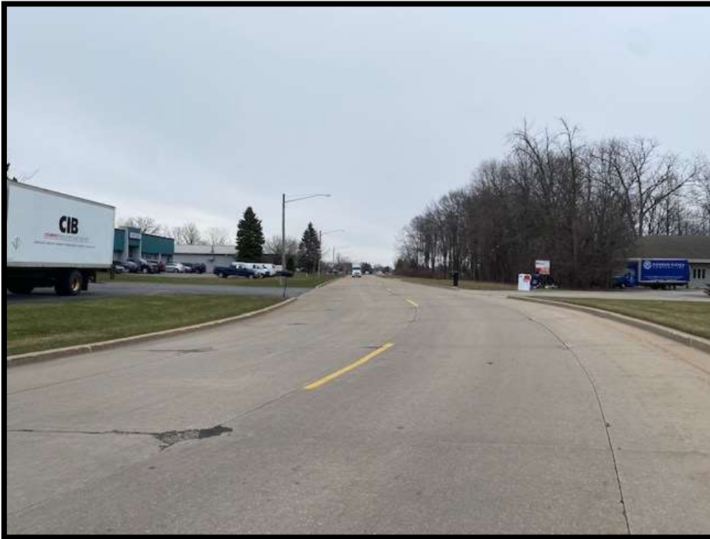
View of Kennedy Avenue, looking easterly from near Station 32
