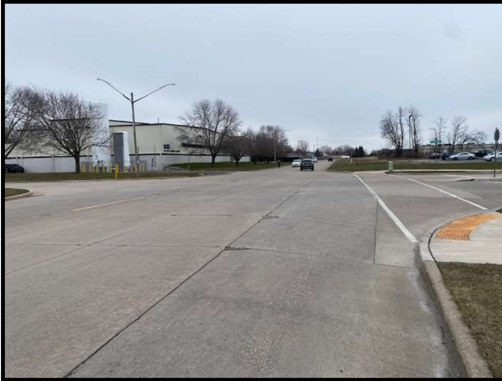
View of Kennedy Avenue, looking easterly from the intersection with Eisenhower Drive (Station 52)
