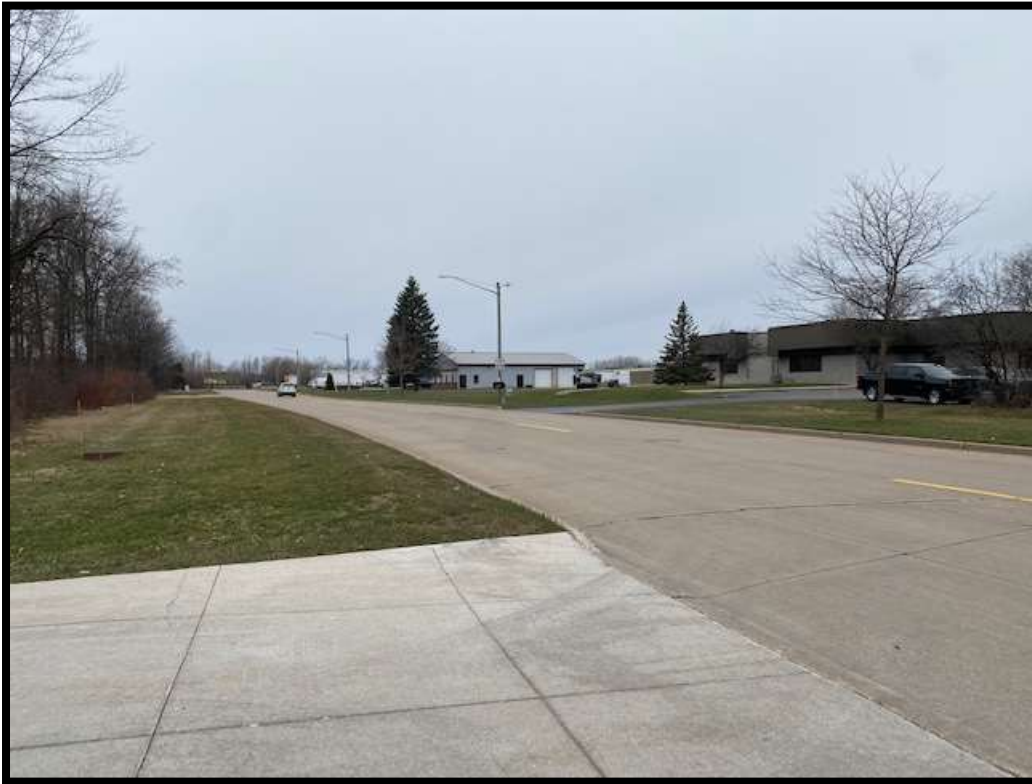
View of Kennedy Avenue, looking westerly from near Station 40
